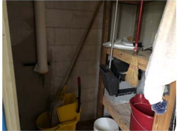
VIEW OF TYPICAL STORAGE CLOSET
