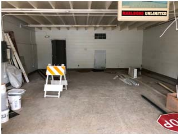
VIEW OF SOUTH RETAIL BAY
