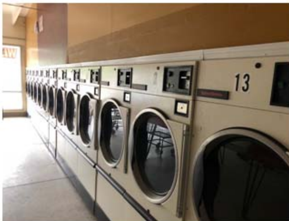
VIEW OF EXISTING LAUNDROMAT EQUIPMENT (WALL)
