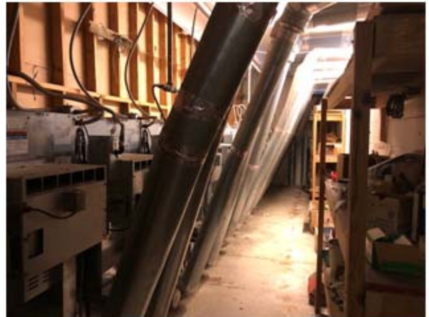
VIEW OF NORTH BAY (REAR STORAGE/MECH AREA)
