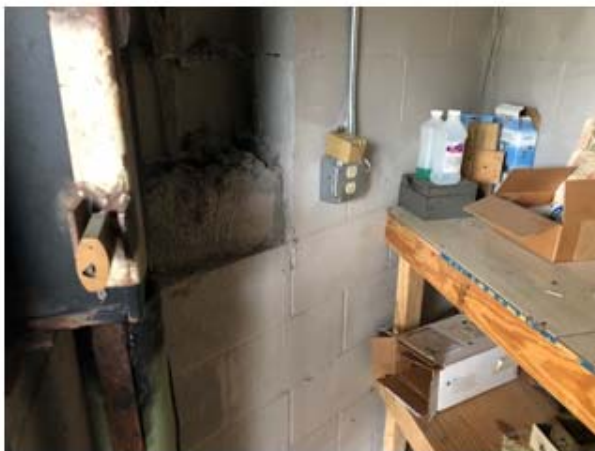
VIEW OF STORAGE ROOM/CHANGE MACHINE (REAR)
